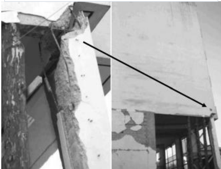
complete diagonal failure of an unreinforced joint
